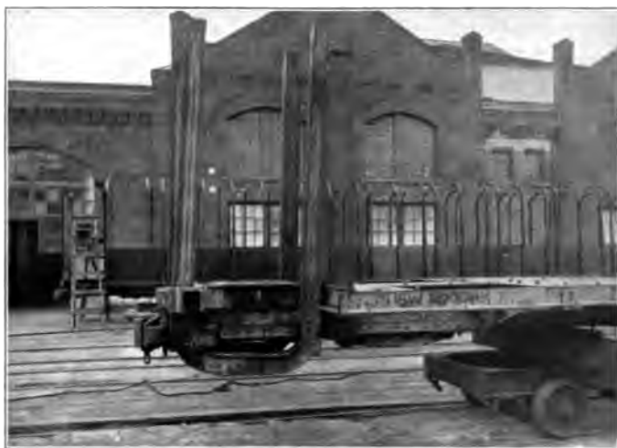
The steel end posts in position, providing strongest possible protection in case of collision
